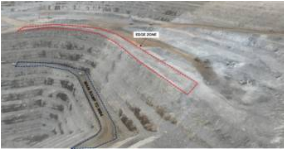
Figure 1. Phase 5 of the WB pit, edge zone and affected ramp area.
