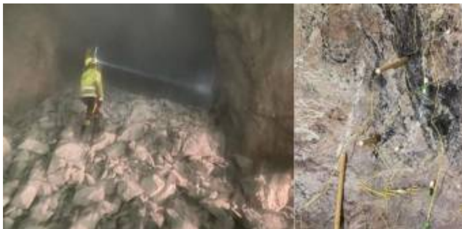
Figure 10. Blast result using the 1st Proposal (left), and wood stick separating the two charges (right).
