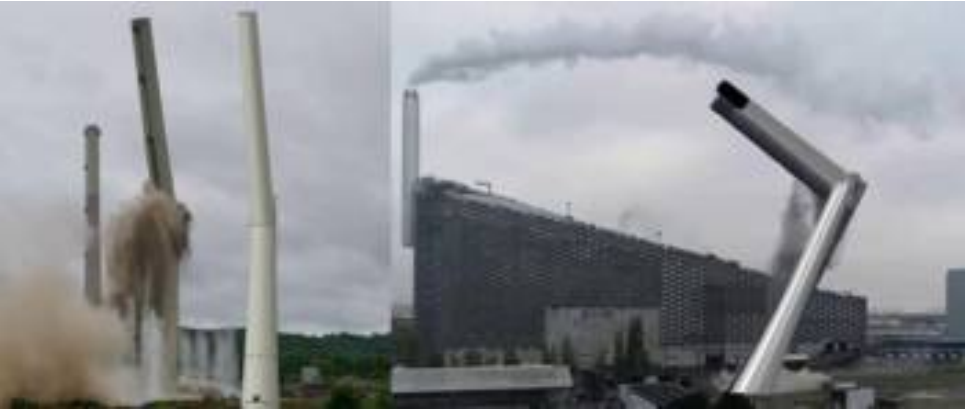
Figure 3. Simulation and real blasting of chimney blast folding in Ens Dorf (left) and Copenhagen (right).
