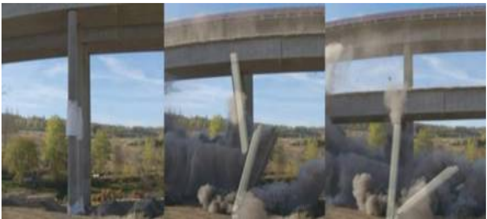
Figure 4. Overlay plot for the blasting of the northeast viaduct 'Landeskroner Weiher'.
