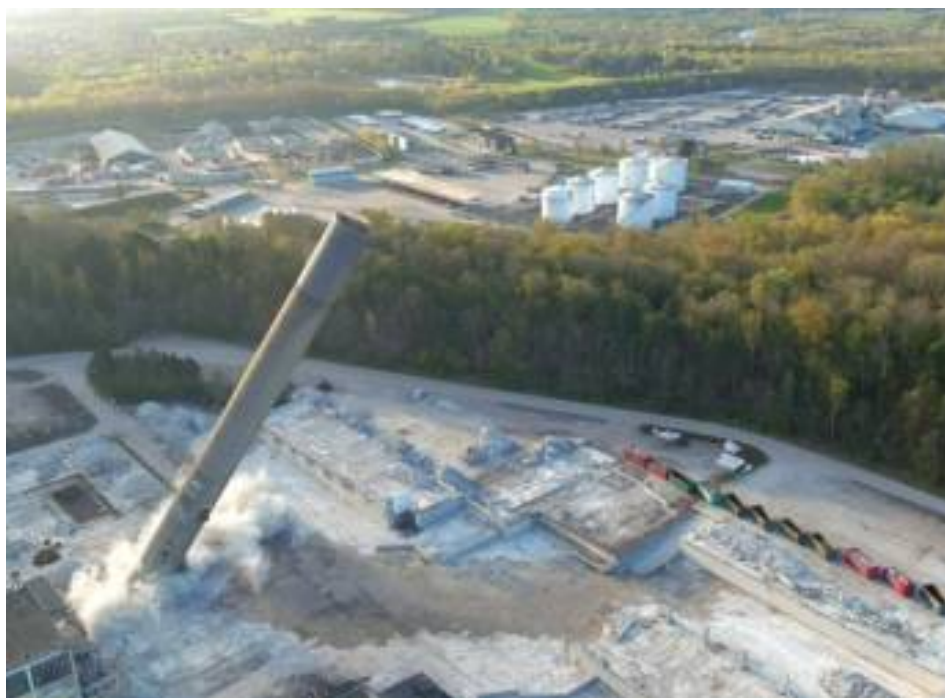
Figure 5. Chimney at Hedehusene, Denmark demolished 30 April 2023.
