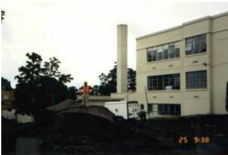
Figure 2. Blasting up 1.5 m of a school. With students inside. St Helens, Oregon, USA. Photo credit: Doug Harding.
