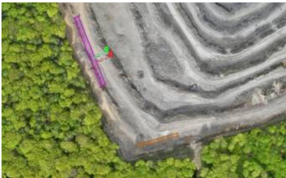
Figure 14. Location of fifth blast comparison according to series of perforating holes.
