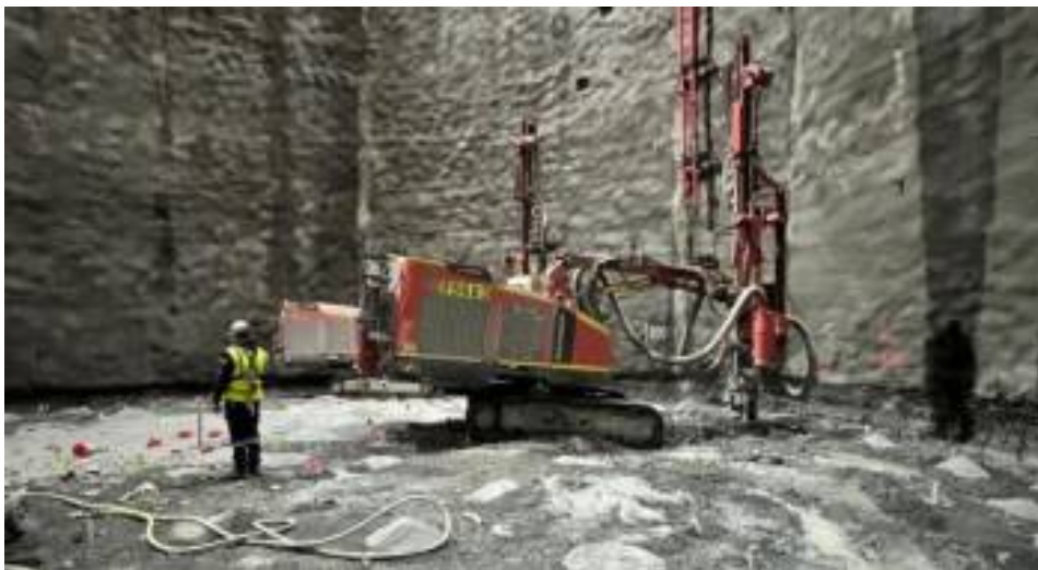
Figure 3. Drilling the blast.
