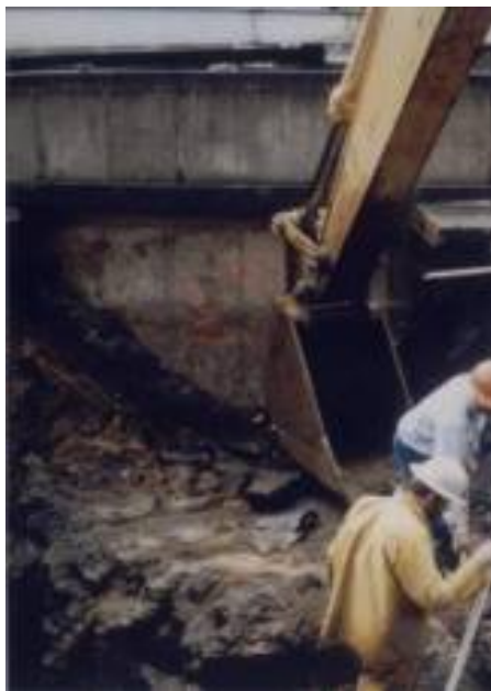
Figure 3. An example of a bench with blastholes being loaded for a poured-to-solid foundation. Blasting to tie in to the sewer tank just behind the excavator bucket (containing stemming material). Sweet Home, Oregon. Photo credit: Bill Parke.
