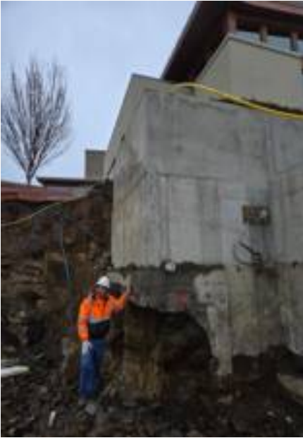
Figure 8. Successful completion. Note oxidized existing joint structure. No damage to existing foundation, no vibration issues, no flyrock.
