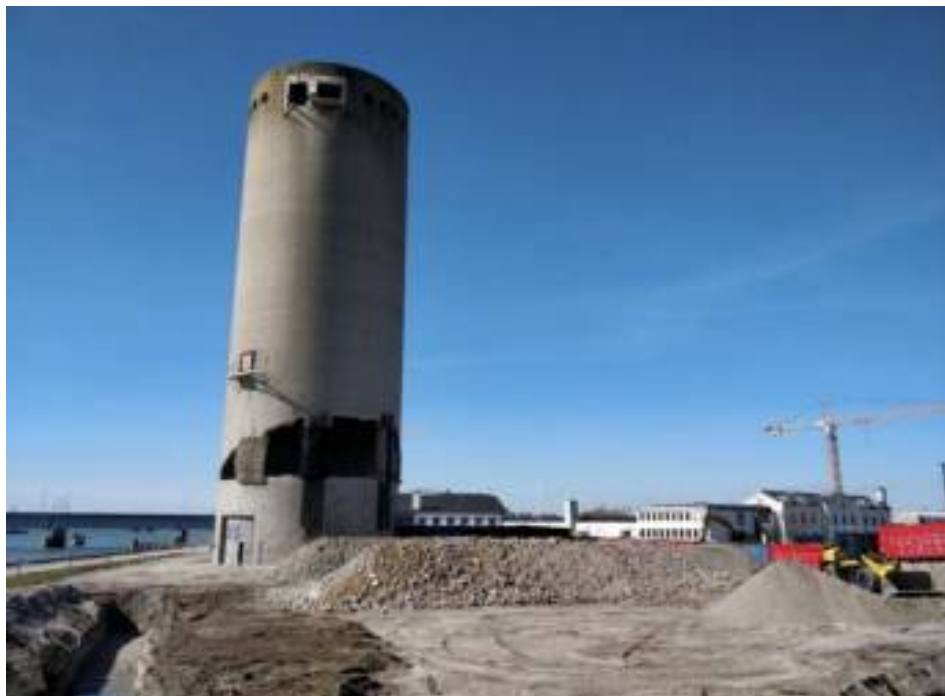
Figure 1. Cement silo at Vordingborg, demolished 6 April 2018.
