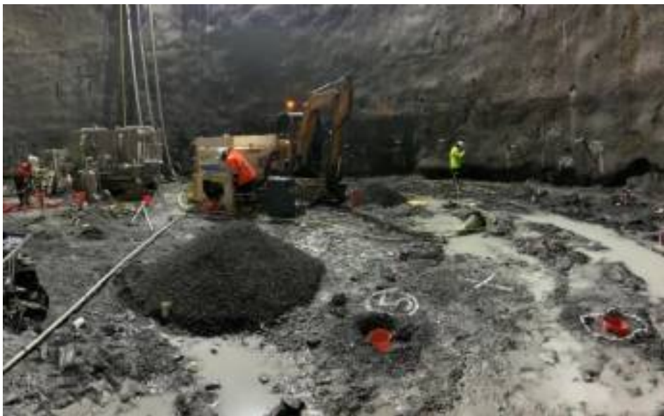
Figure 5. Loading shot at Level 46 in Marica shaft.
