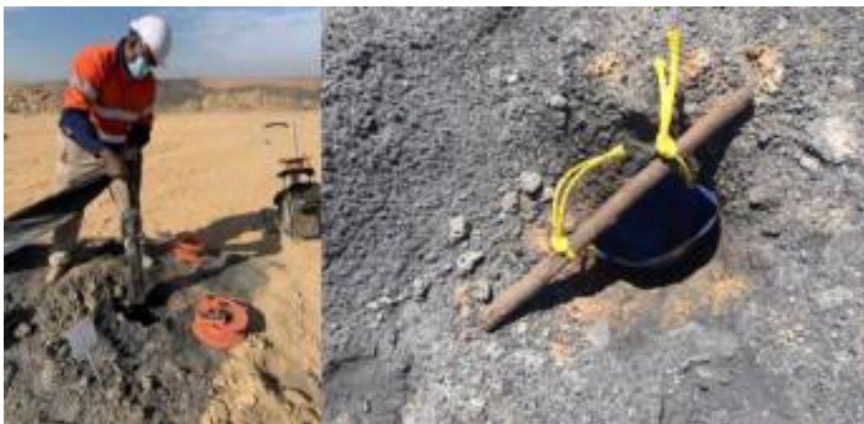
Figure 8. Photographs showing a sleeve being lowered into the hole and a sleeve ready to be charged Stenzel (2021, 2025).
