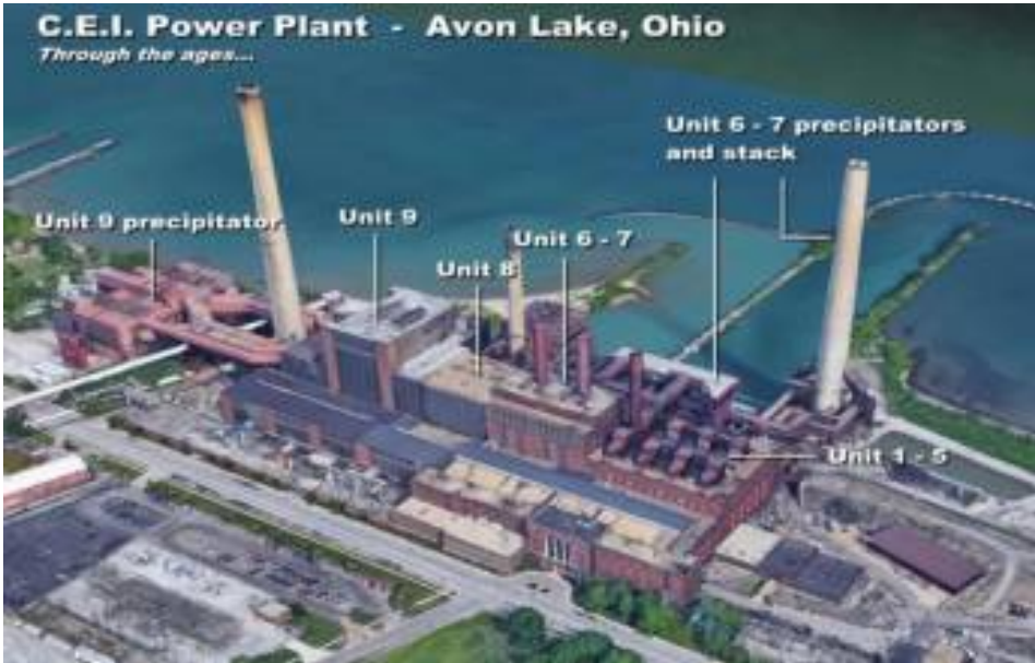
Figure 1. Avon Lake power plant prior to demolition.
