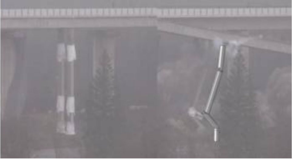
Figure 5. Overlay plot for the blasting of the southwest viaduct 'Landeskroner Weiher'.
