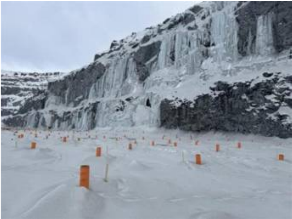
Figure 10. Ice hanging on the pit high wall creates a hazard.
