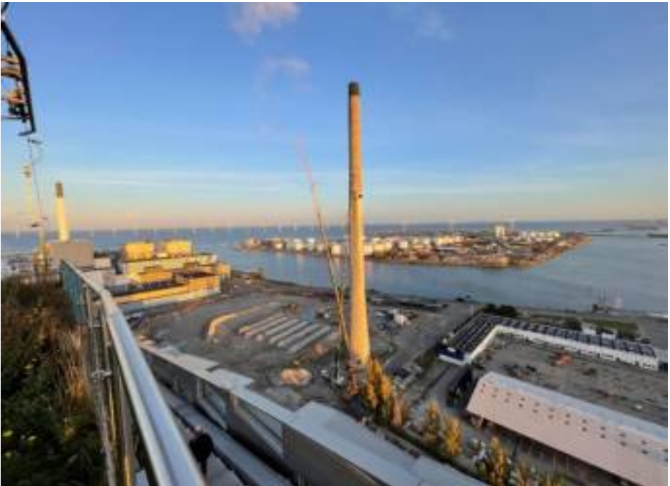
Figure 3. The chimney at Amager Resource Centre demolished 31 October 2021.
