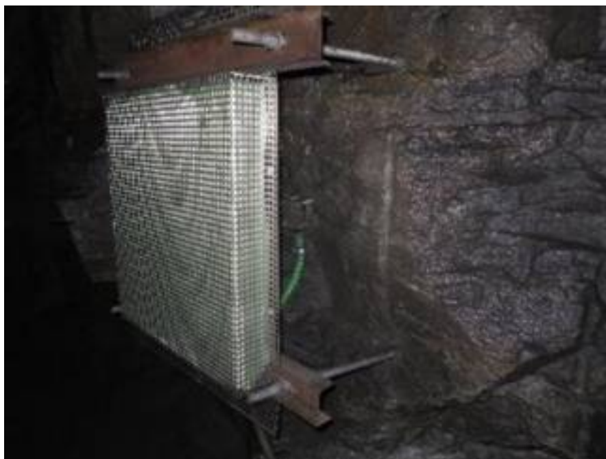
Figure 12. The complete cage mounted in front of Sensor 3.
