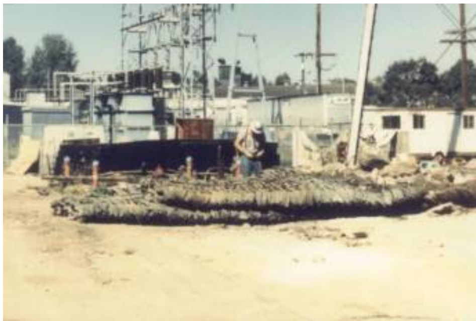
Figure 4. Complex industrial site work, trenching and foundations with multiple structures both overhead and in the ground. St. Helens, Oregon. Photo credit: Bill Parke.
