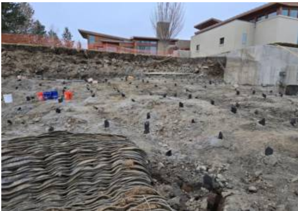
Figure 6. Wine cellar, tying in to foundation of structure to right, house 12 metres beyond. Blasting mats used to limit flyrock. Looking north. Photo credit: Jerry Wallace.
