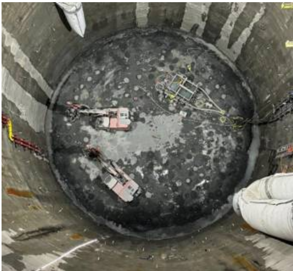
Figure 4. Two drills operating in the shaft.
